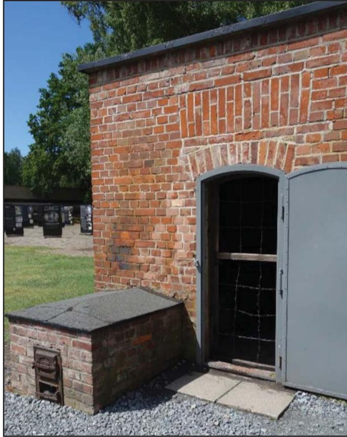
*The front of the Stutthof delousing chamber, as can be seen today. Note the heating oven next to the door. This provided heat to a shelf on the inside of the delousing chamber to activate the Zyklon-B pellets which were laid down on the shelf."*
