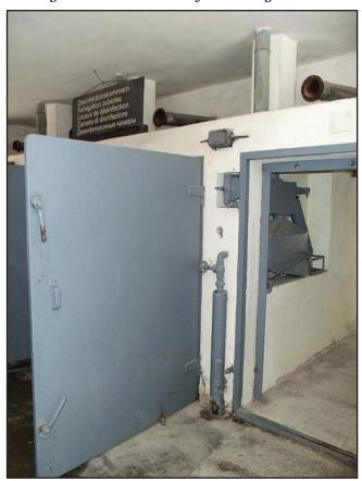
Below: The rear (outside) of the Dachau disinfestation chambers. The double doors on both ends of the disinfestation chambers were necessary to keep clean clothes separate from the contaminated ones—dirty clothes were put in on one side, and clean ones taken out the other—just like in Auschwitz.
