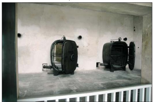
Below: Prisoners at Auschwitz working in one of the larger clothing disinfestation chambers in the camp. They worked in much the same way as the autoclaves, with "dirty" and "clean" sides. The peepholes in the doors could be closed by raising the flap and blocking it with a catch. These were opened at the end of a disinfestation cycle to allow fresh air to enter as soon as the extractor fans were switched on. Photographs from the Auschwitz museum archive.
